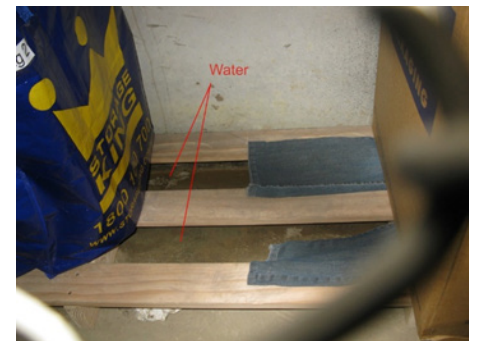
Figure 3 – Storage cage with water flowing in the drain at the wall-floor junction
