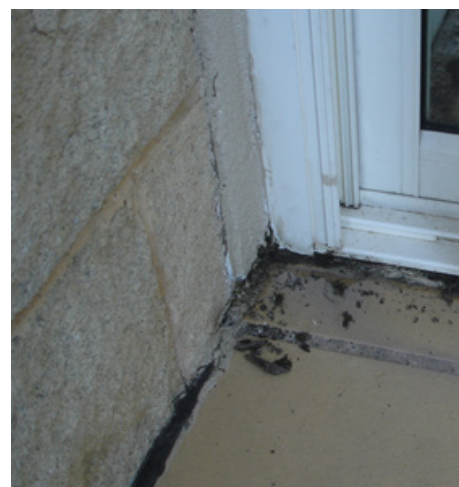
Figure 2 - Windowsill located directly onto level of deck
