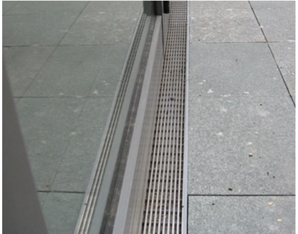
Figure 4 – Grate drain installed across a doorway
