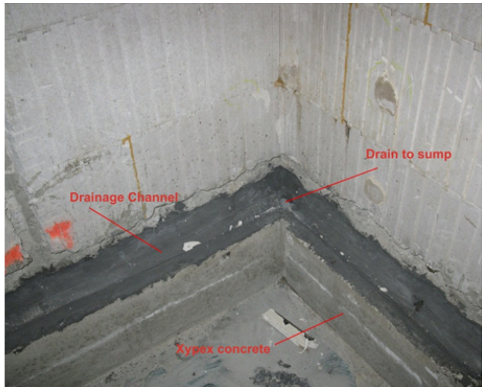
Figure 5 – Basement before installation of the plasterboard wall supported on metal battens
