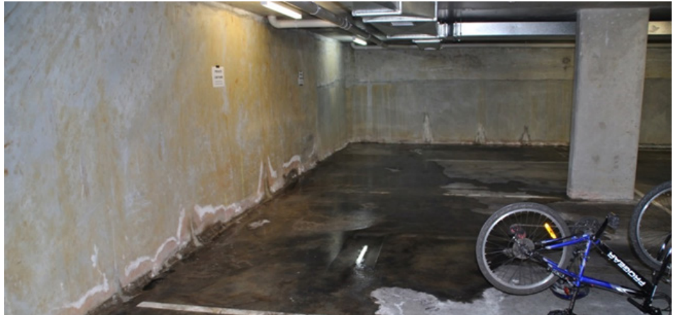
Figure 1 - Flooding of the floor of a car park basement by leaking at the floor-wall junction
