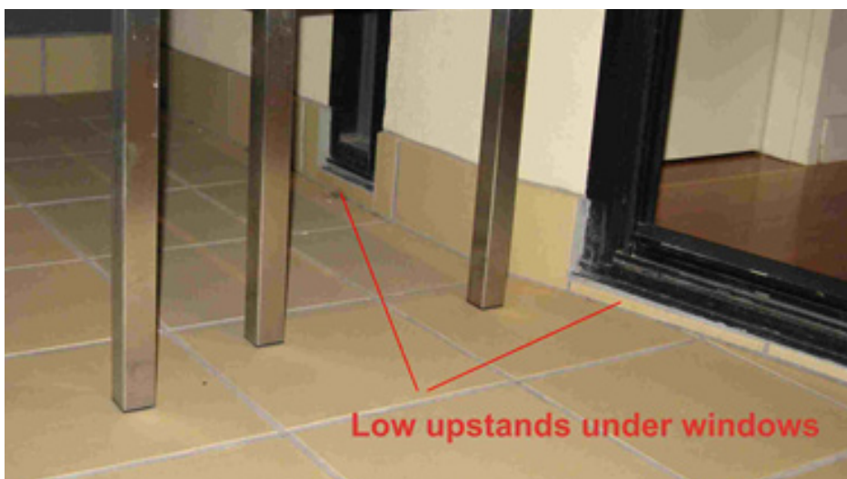
Figure 3 – Low up-stands under window
