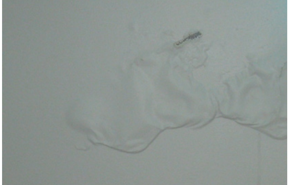
Figure 4 – Blistering of paint finish by water vapour
